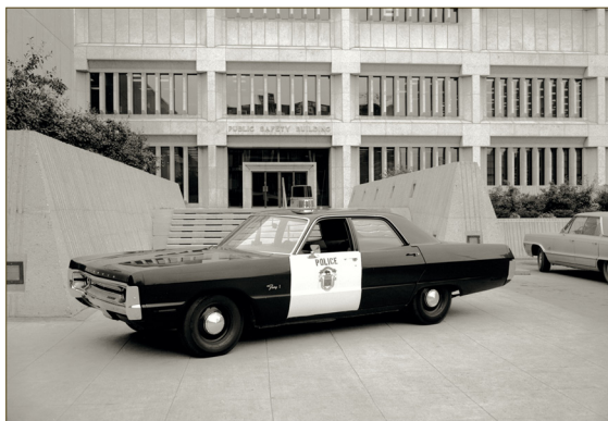
New Winnipeg Police Cruiser Car (1971 Plymouth Fury II) parked outside the front entrance of the Public Safety Building at 151 Princess Street, Winnipeg, 1971c
