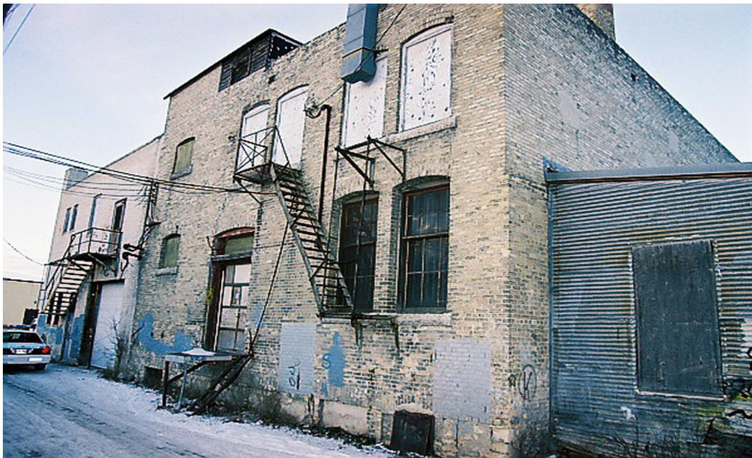
Rear View of the warehouse complex
