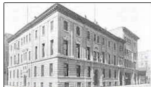
Central Police Station ("A" Division) Rupert Ave. & Louise St.
