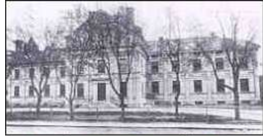
Vaughan Street Detention Home
