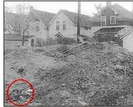
George Smith's clothing (circled) at the rear of a house under construction.
