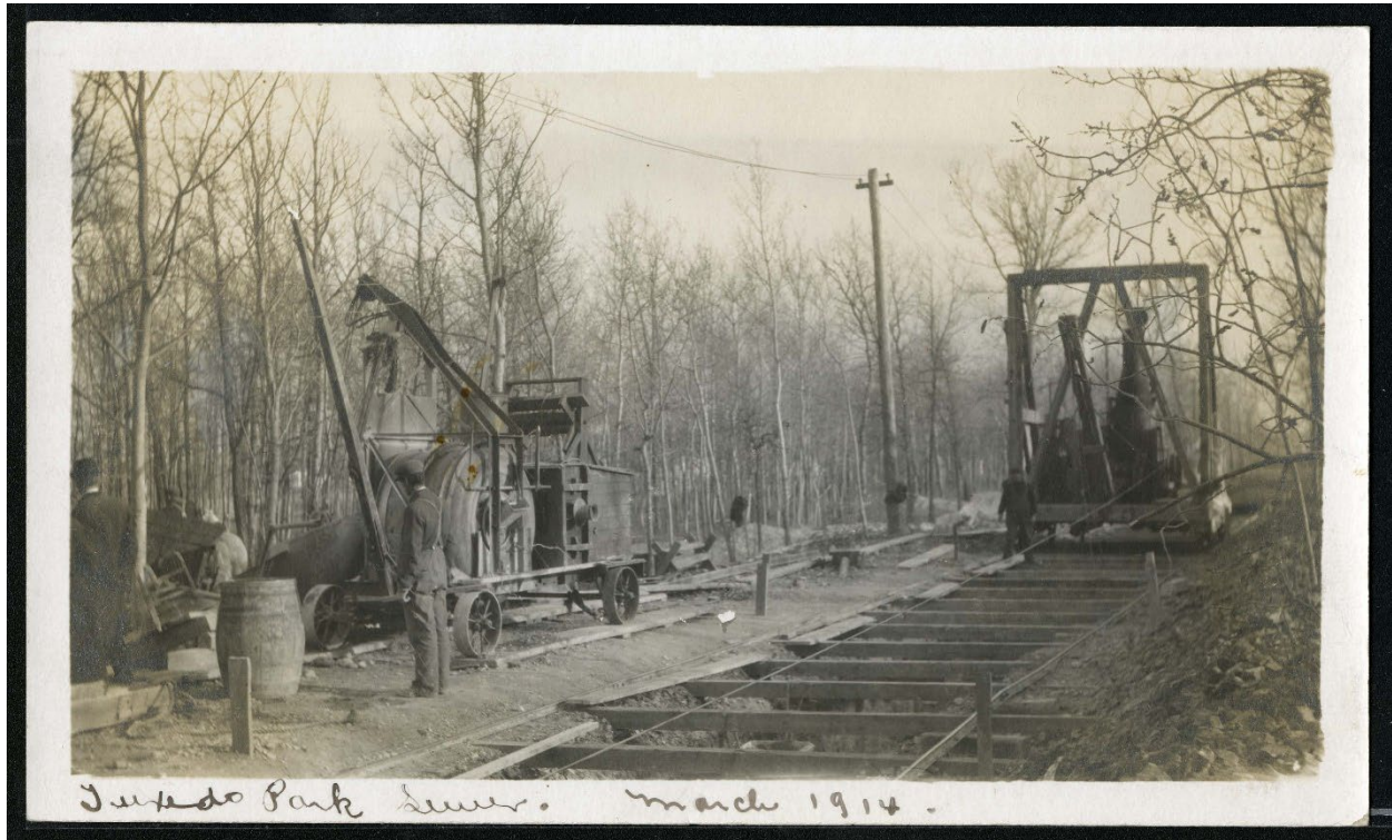
Building Tuxedo Park Sewer, March 1914. City of Winnipeg Archives, Morris Block Collection
