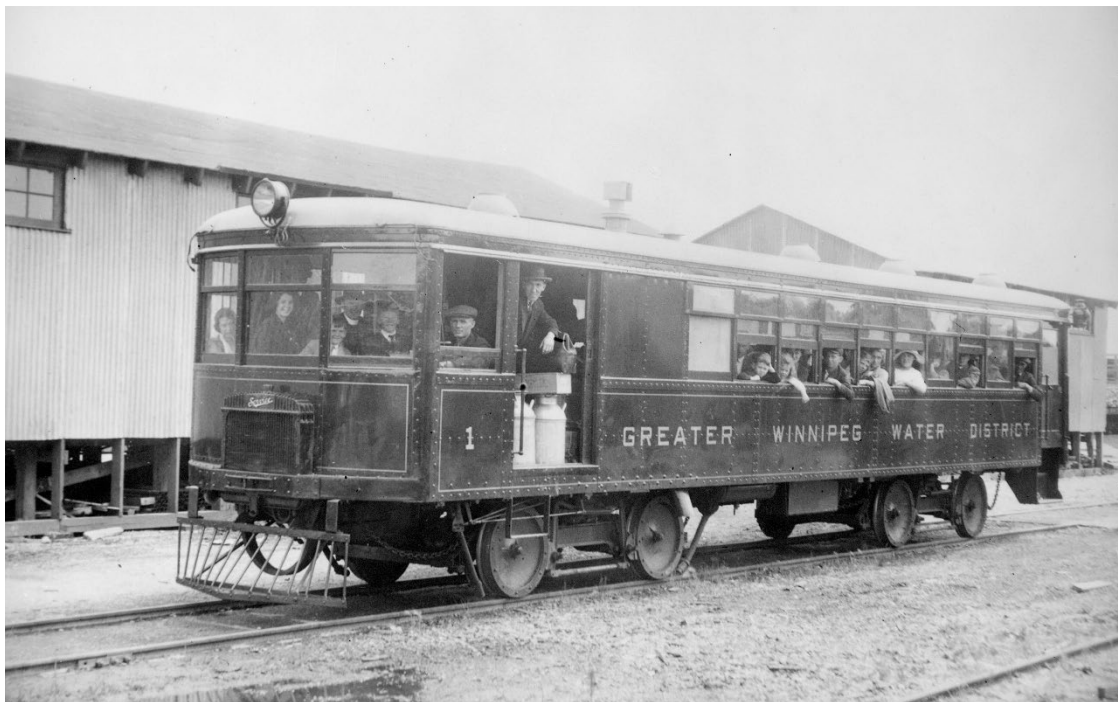
Greater Winnipeg Water Works railway car. City of Winnipeg Archives
