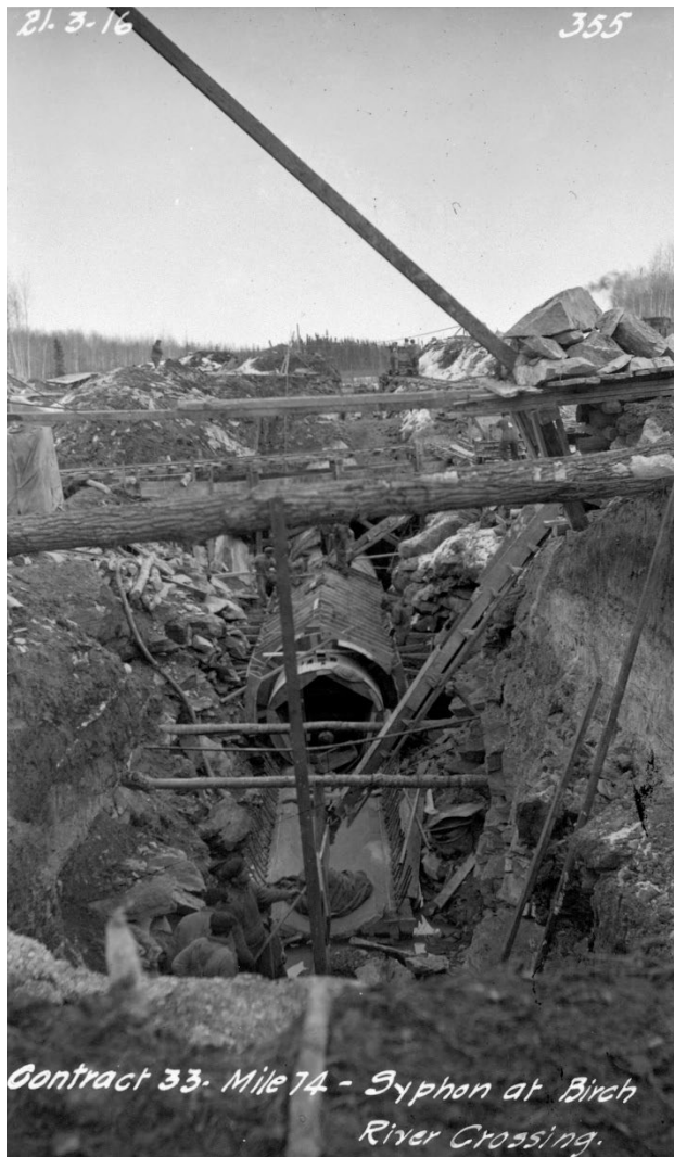
GWWD Syphon at Birch River Crossing, March 21, 1916
